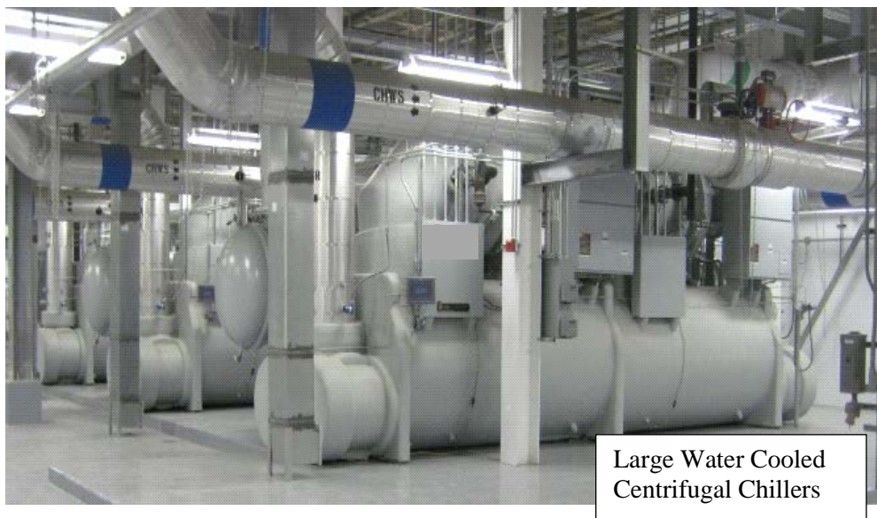
Figure 9-3: Large Water Cooled Chillers in a Mechanical Equipment Room
