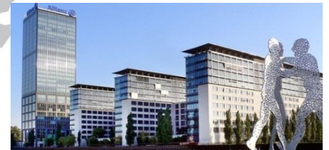
Office complex, 4220 kW
