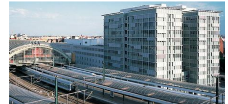
Railway station 1,250 kW
